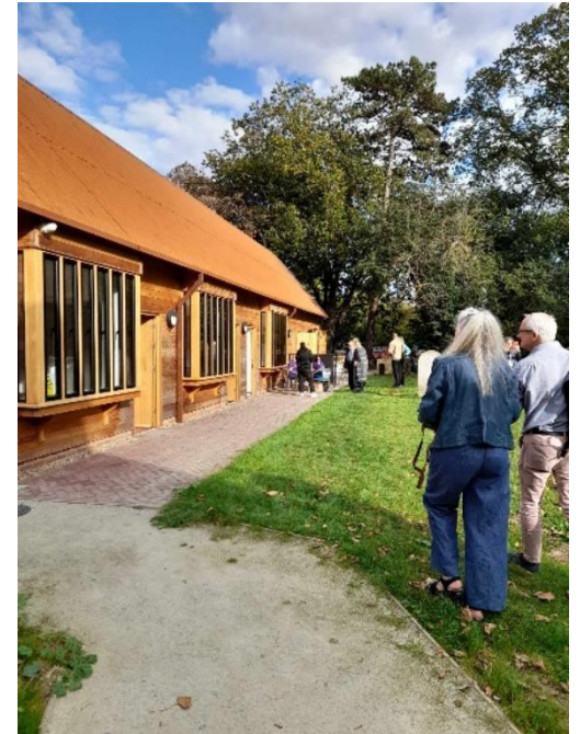
The newly constructed community arts centre at Murston Heart.
